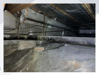
Typically, crawlspaces are unheated spaces and may be ventilated with small vents that penetrate the foundation walls to promote a small amount of airflow through the crawlspace. Crawlspace foundations are less expensive than full basements because they require less excavation and less foundation wall material and labor to build. Crawl spaces also used if soil is tough to dig excavate.
