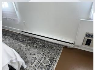
Unlike forced-air heating systems, baseboard heaters don't blow air, which means less dust, allergens, and pet dander being blown around. Baseboard heaters eliminate the need to route air ducts through the house. You also won't hear a furnace firing or rushing air through ductwork and vents. Electric baseboards give you nice, gentle heat without any noise.
