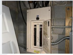
the magnetic force of the solenoid or strip becomes strong enough to trigger a metal lever in the switch mechanism, which breaks the current; other types have metal strips which can bend, triggering the switch and breaking the connection. To restore power, flip the switch back on, which reconnects the circuit.
