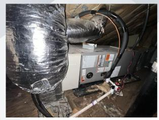
When air is lost because of duct leaks, energy used to heat or cool your house is wasted. If ducts are contained inside your home, the lost energy might be contained within your home, but it might be released into wall cavities and crawl spaces, not living areas whose temperature you want to regulate. If some ductwork is outside, make sure that insulation is secure and tight to help air passing through the ducts maintain temperature until the air reaches living areas.
